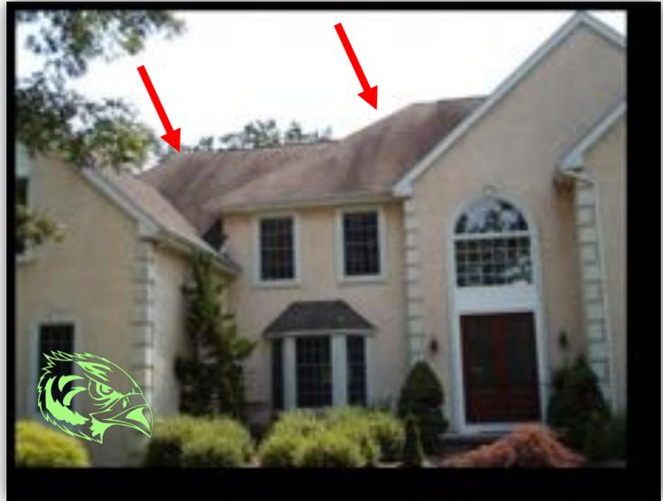
**Roof algae** are the first wave in a succession of organisms that can colonize and ultimately undermine a roof. The algae can eventually team up with a fungus to form lichen. Moss follows, building a small layer of soil that might catch seeds from bird droppings. By the time grass sprouts between the shingles, it's past time for a new roof. **The process can take years.**
